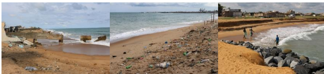
Fig. 31. Visiting Cotonou's coastline. On the left it is shown how erosion has destroyed a building that was educating future mothers, in the middle the plastic problem is illustrated with on the background the port of Cotonou in full development. On the right some local fishermen are busy working. (Photo@K. Baetens and M.L. Susini Ondafe)
