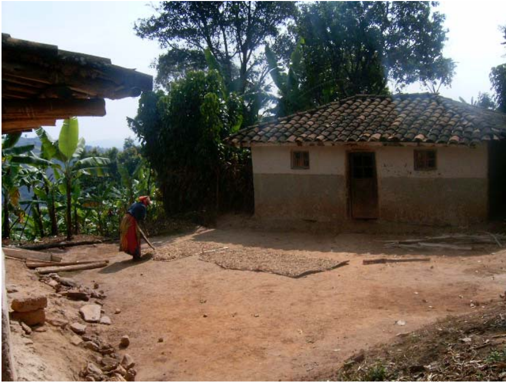
Fig. 17: The majority of the houses are built with mud out of bricks and cooked tiles in Mutana and Rukoma hills
